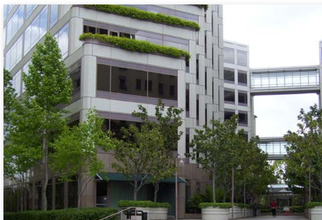
PRUNING FOR BUILDING CLEARANCE
